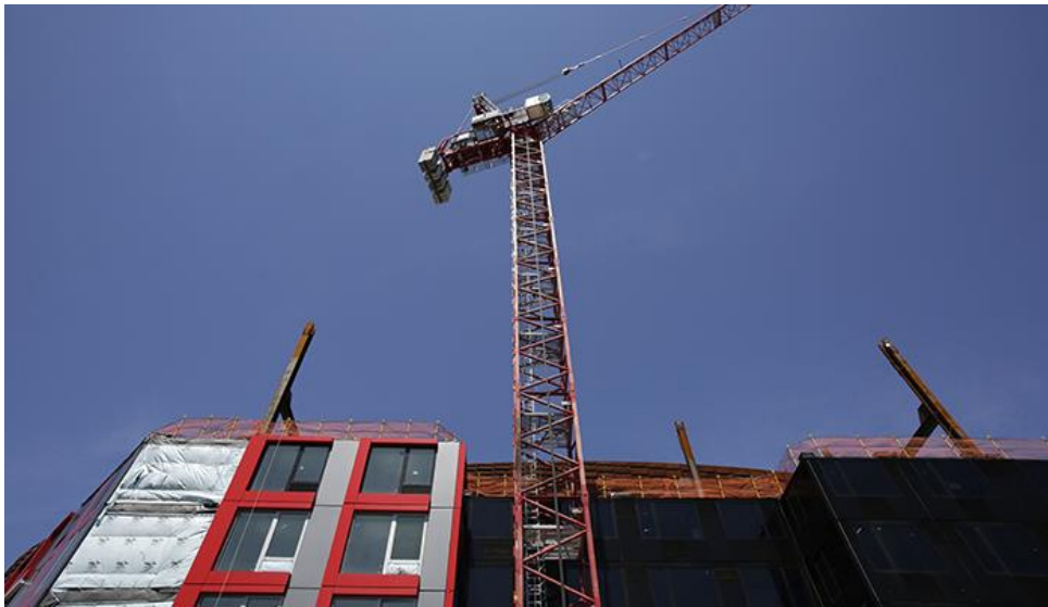
Construction in Brooklyn. (AP Photo/Mark Lennihan)
